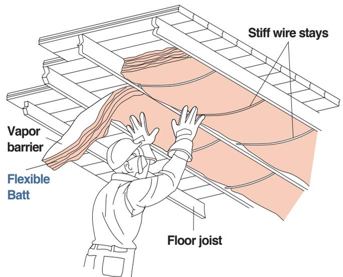
Figure 3-20 - Installing batts in basement ceiling.
