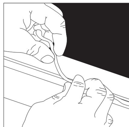
1. Wearing heavy gloves, remove broken pane. Pull out old glazier's points with needle-nose pliers. (Glazier's points come in two styles: diamond, shown here or push type, step 4.)
