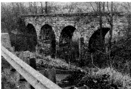
Figure 17. Valley Railroad bridge, Augusta County.
